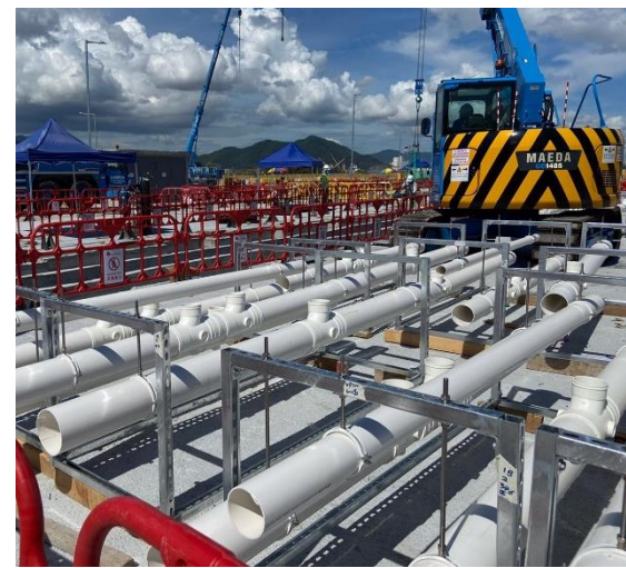
Prefabricated Drainage pipe modules to be installed
