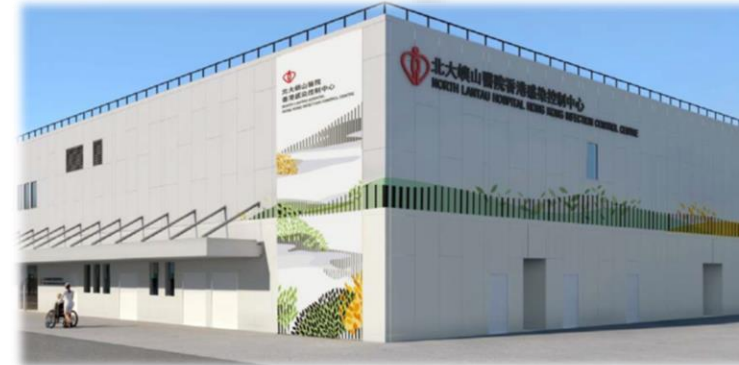
North Lantau Hospital Hong Kong Infection Control Centre
