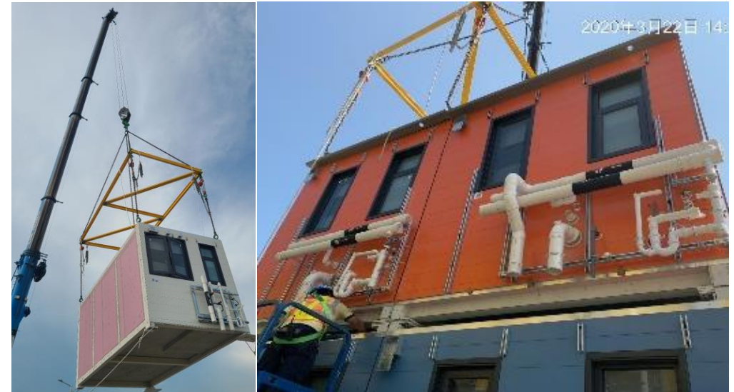
Module pre-installations in factory or on-site
