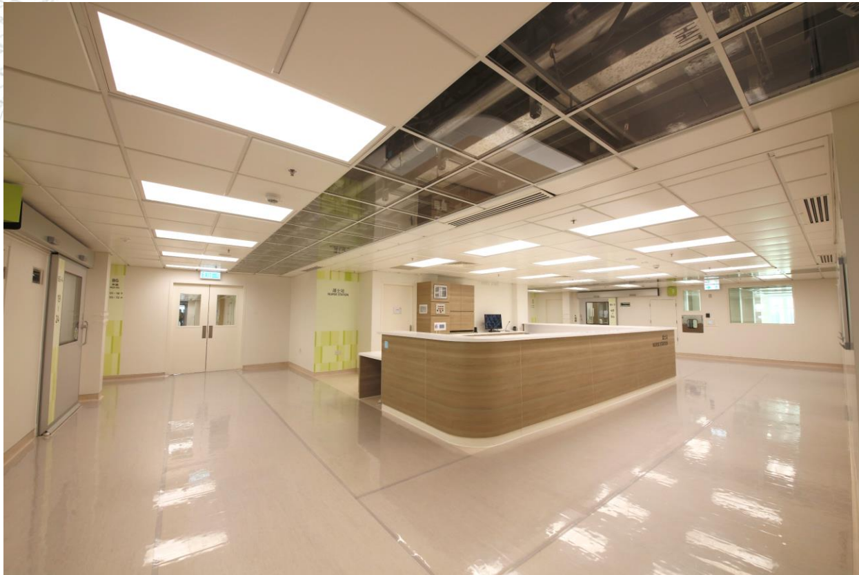
MiMEP modules are installed with transparent ceiling panels in wards
