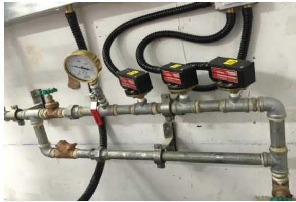
Pressure Switch Assembly for Sprinkler System
