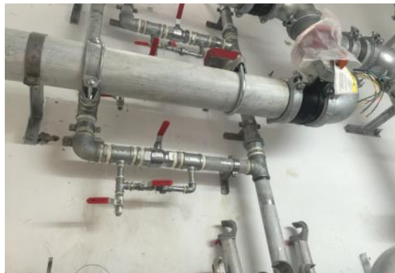
Sprinkler Test and Drain Facilities
