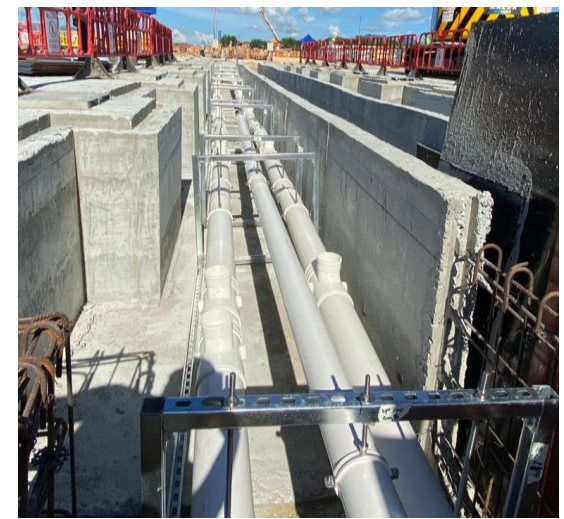
Installed drainage pipe modules installed in pre-casted trench
