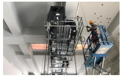
Ready For Installation
